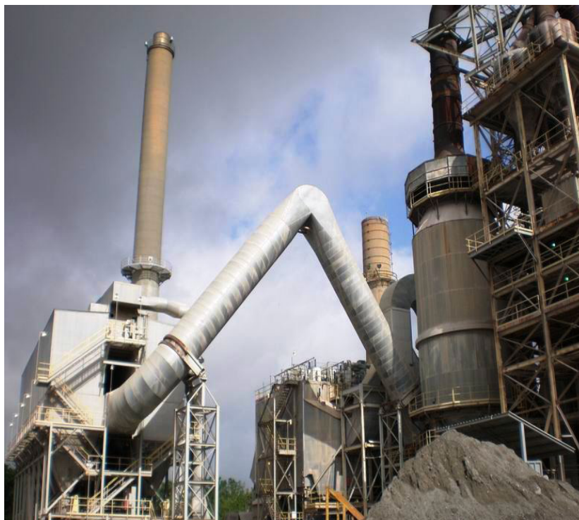
Figure 3: View of the Midwestern Cement Kiln
